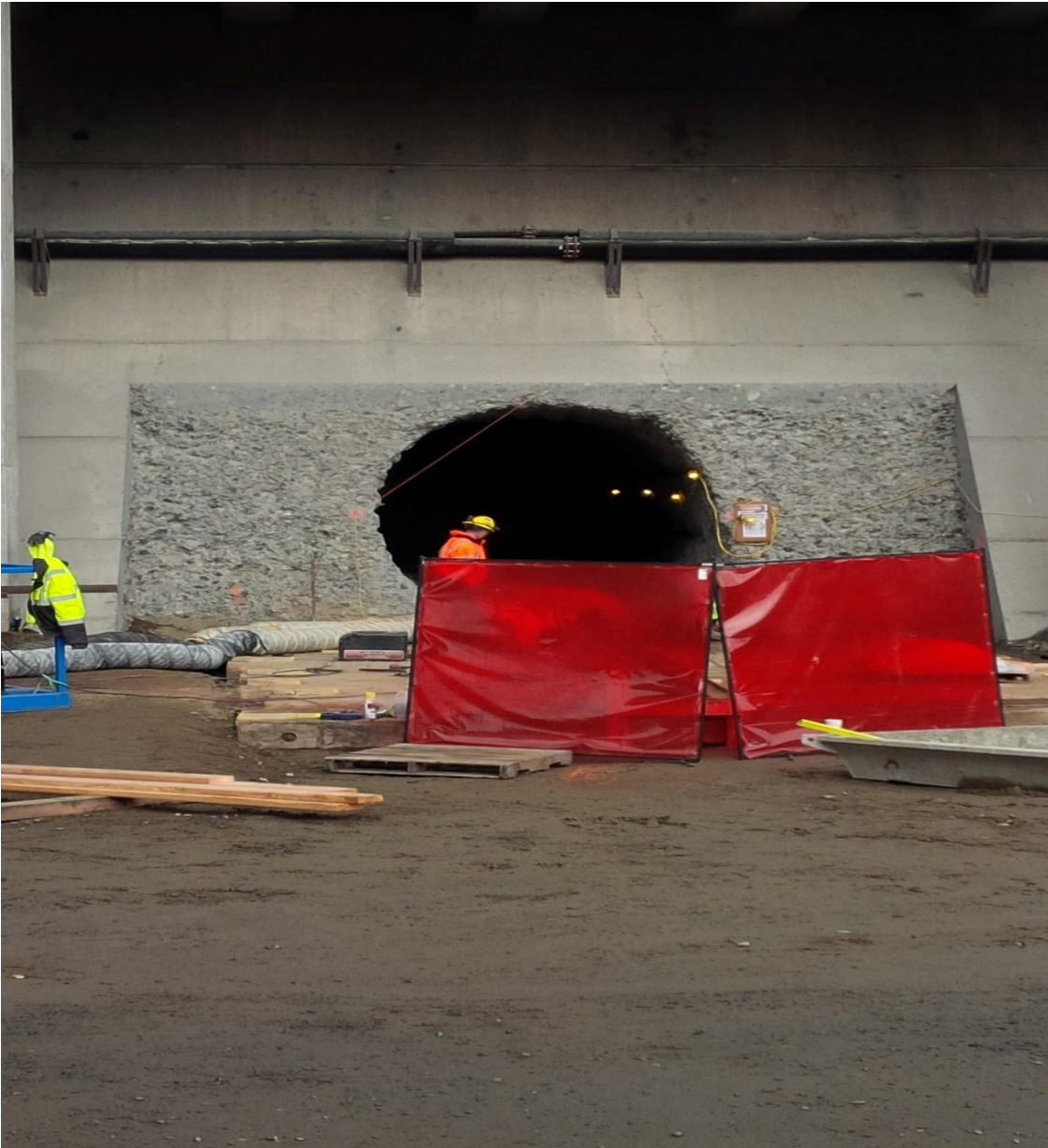
Prepping slide to insert 10' pipe in dam.
